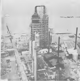
ONE OF the most photographed units in this refinery or any other is undoubtedly the cat cracker. It is "shot" during the day from many angles, at night, at Christmas-time bedecked with brightly colored bulbs, and even when it is undergoing a general inspection. Here is a different shot. It's taken from the flare stack UN DI e plantanan na fotografia den e refinaria di cualkier otro sin dula ta e cat cracker. Den dia e ta wordu sacá for di varios punto, anochi, durante dianan di Tawata ora e ta dora cu centenas di luznan di color y hasta ora e ta bao pa inspeccion general. Aki sinembargo, nos tin un retrato for di un punto stranjo. E ta saca for di e flare stack
